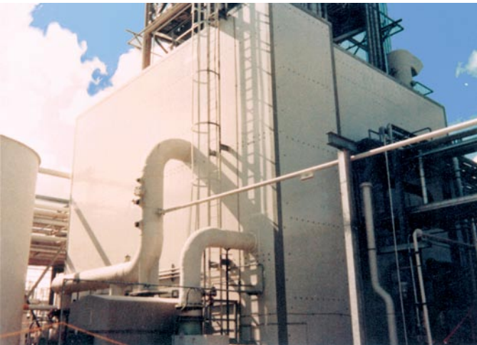
Airtight enclosure for Dow Chemical protects workers in adjacent areas against accidental escape of phosgene gas.
