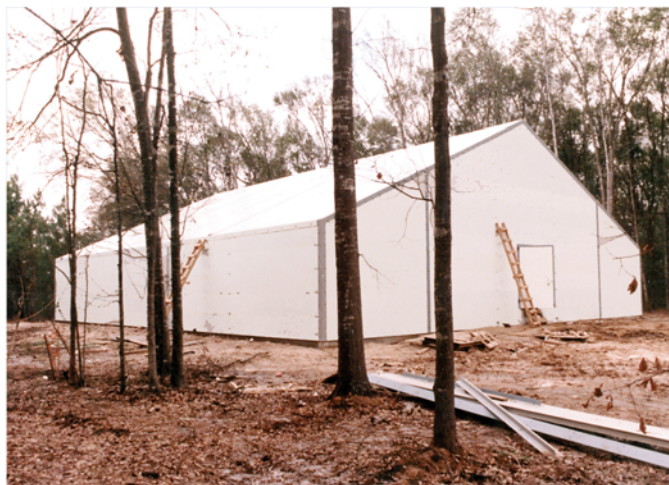
Compaq Computer chose a foam core panel building to assure RF/EMI compliance for attenuation.
